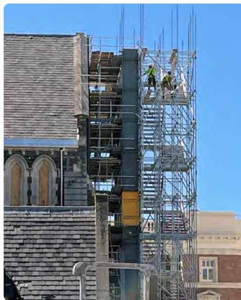
Safety scaffolding provides stone masons access to the damaged wall. Credit CCRL
