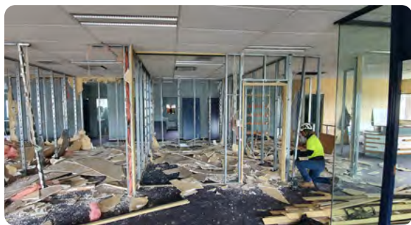
The old temporary partitions being deconstructed. Credit: Integrus.
