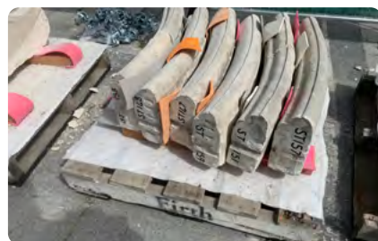
Limestone profiles numbered and stacked. Credit: CCRL
